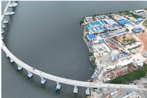
Rapid Transit System (RTS) Link, Johor (Perenggan 162)
